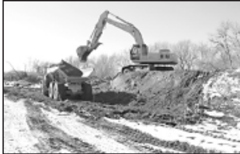
Early construction of the holes west of the South Platte River.
